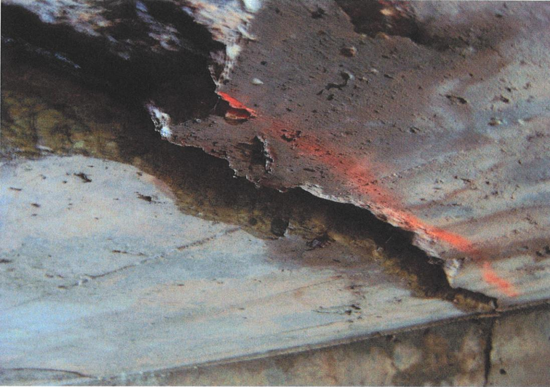
1" crack in bottom of top slab
