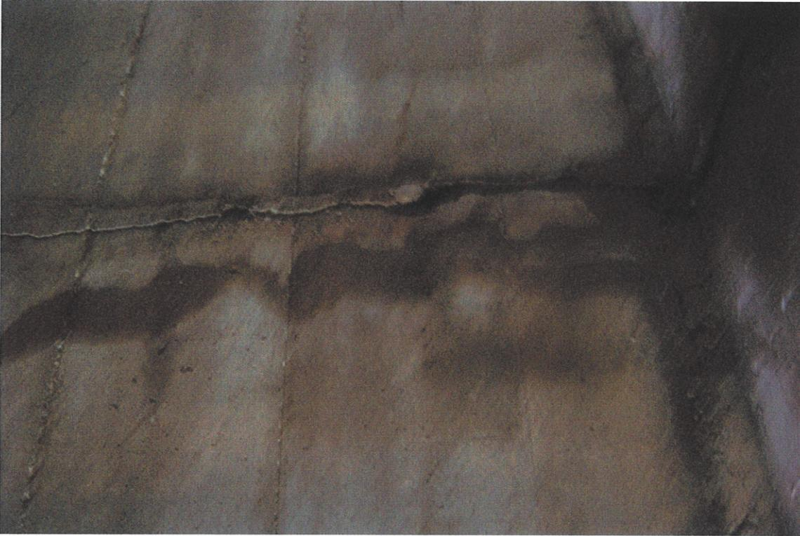
1/4" - 1/2" crack in back wall (typical)
