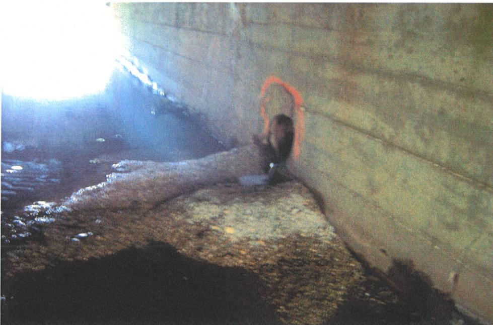
Pipe carrying storm water has failed, allowing rock and sediment to filter in, creating a void in the roadway above.
